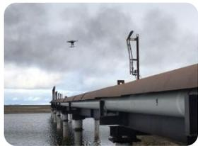
Avitas Systems, a GE subsidiary based in Boston, is now using drones and robots to automate the inspection of infrastructure such as pipelines, power lines, and transportation systems. The company is using off-the-shelf machine-learning technology from Nvidia to guide the check-ups, and to automatically identify anomalies in the data collected.
