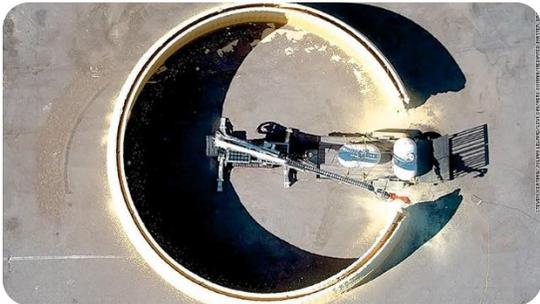
Researchers from the Massachusetts Institute of Technology have created a robotic system that built the basic structure of a building in less than 14 hours. The dome-like structure is 50 feet in diameter and 12 feet high.
